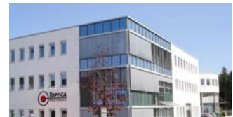
10 years TOPTICA – company building in Graefelfing (Munich)
